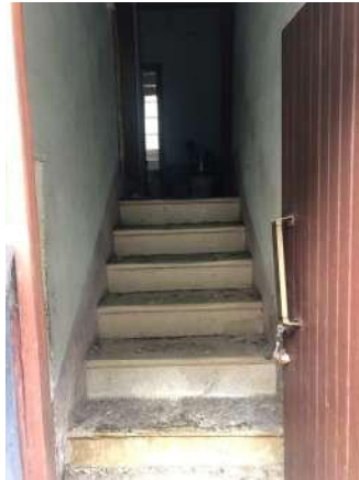
Entrance hall whit stairs
